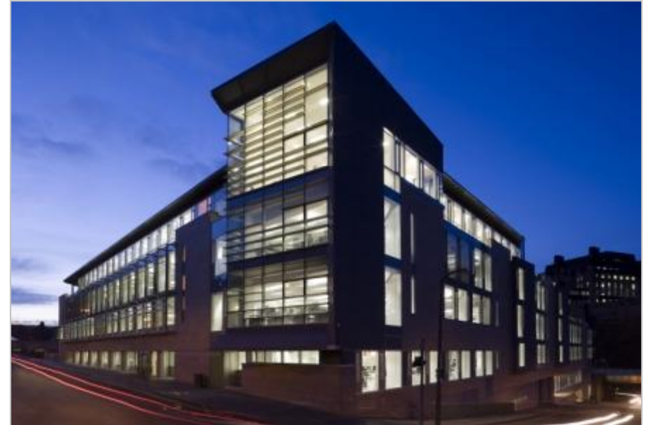
Council headquarters, East Market Street
